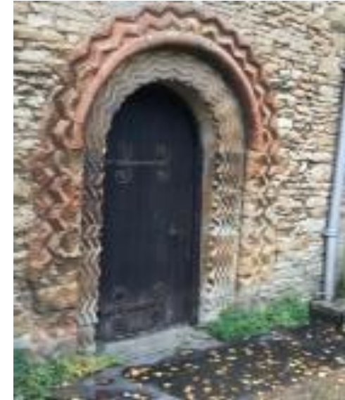
Norman door, south elevation
